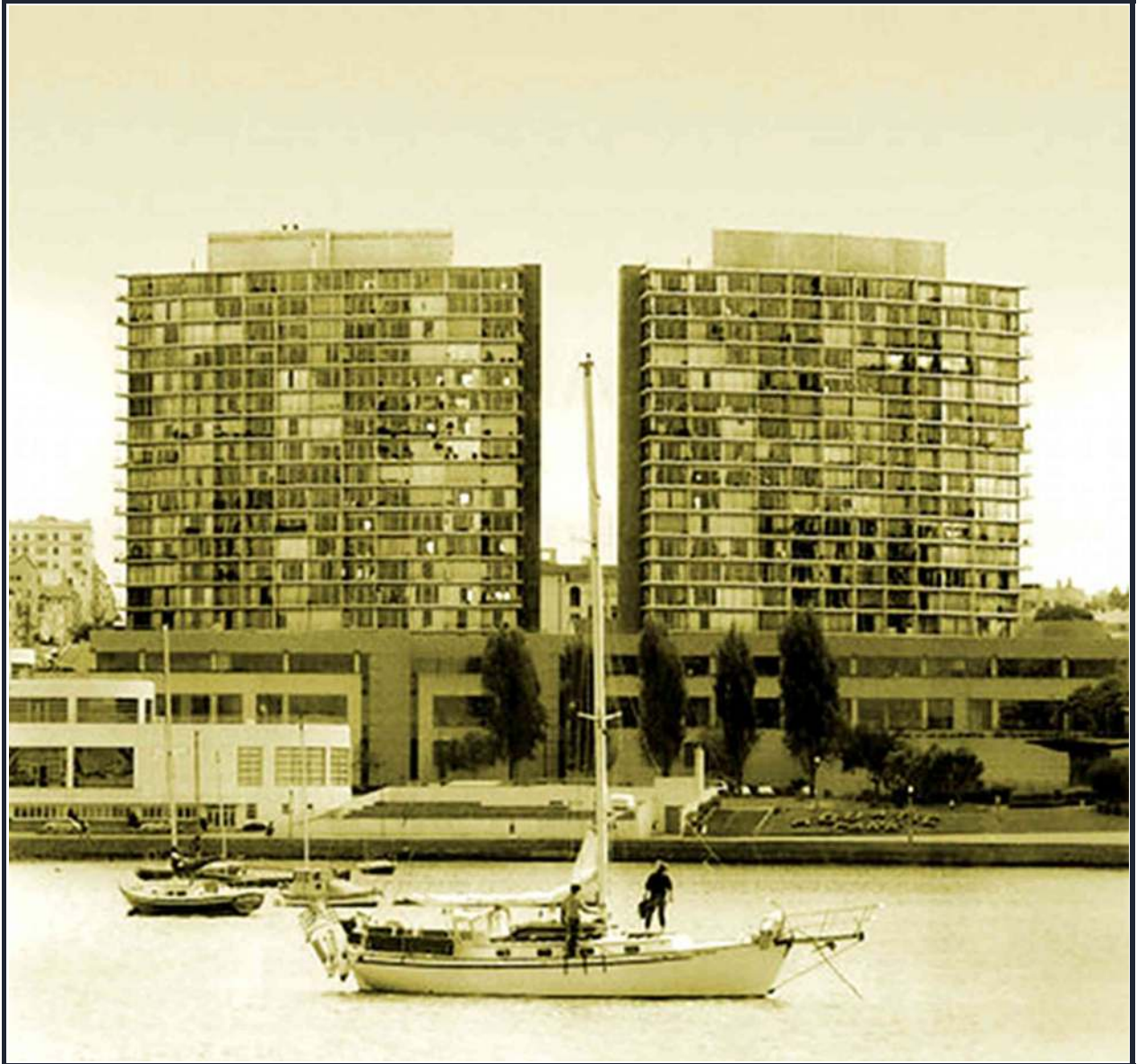
Figure 2: Fontana Residential Complex, San Francisco
