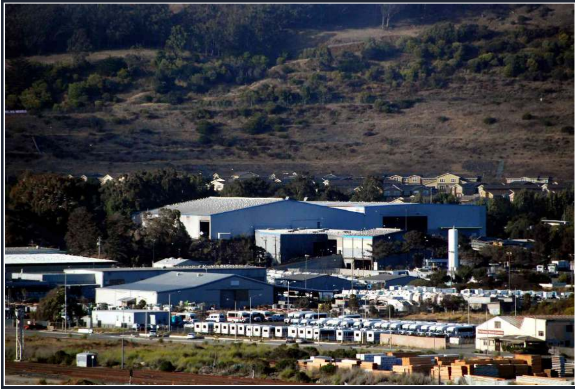
Figure 32: Discharge of Odor
